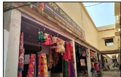
Transit house used as market complex at Jajpur Municipality
